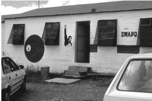
Former SWAPO office in the „Ovambo compound“ Katutura
